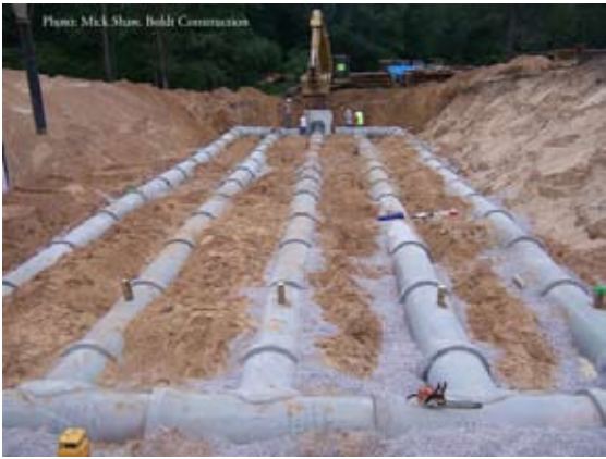
Completed earth tube array
