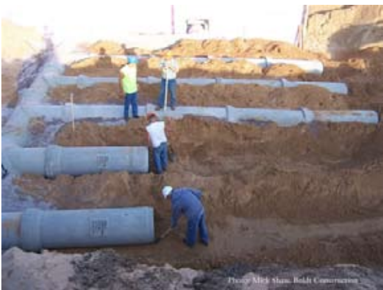
Workers make sure tubes are level and aligned correctly
